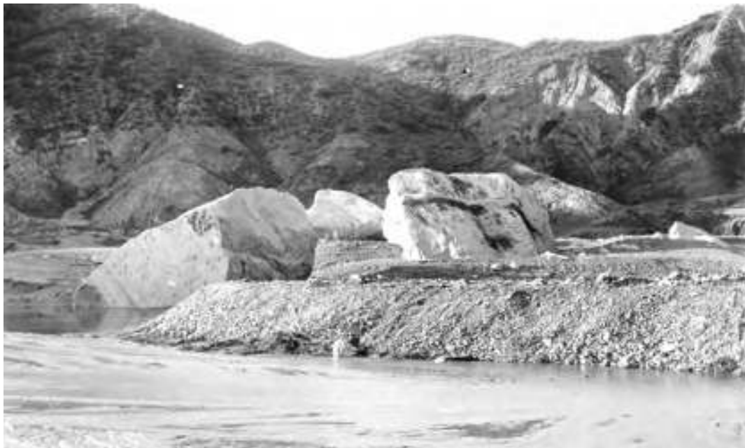
Figure 32. Ground view of Blocks 44, 27 and 43 resting upon a flood outwash terrace of schist detritus, with an average grain size of 10 inches. These blocks were likely freighted upon this extensive blanket of detritus, which emanated from the east abutment landslide. The token cut-off trench beneath the dam's right abutment is seen running diagonally across Block 43 (at right). Photo from the Lee Collection, U.C. Water Resources Center Archives.
