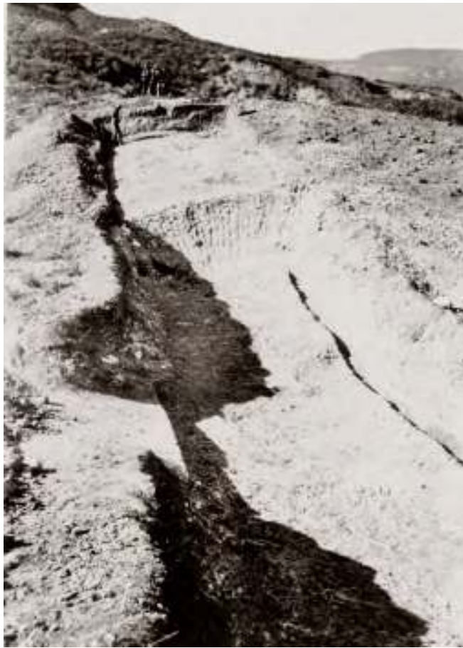
Figure 6. Keyway excavation in the Vasquez conglomerate cut by steam shovel for the dam's dike section, which extended about 600 feet northwest of the right abutment crest. Photo taken from Lippincott collection, U.C. Water Resources Center Archives.
