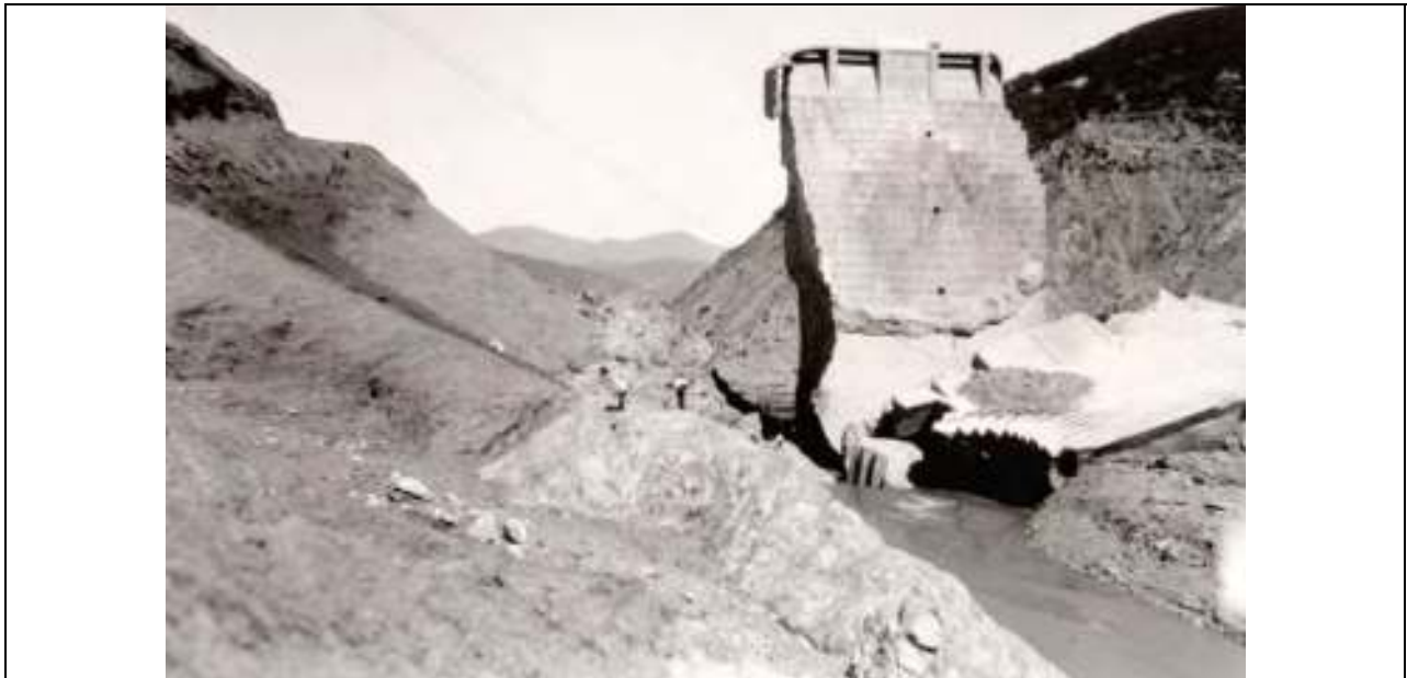
Figure 41. View of San Francisquito fault contact, between the Vasquez sandstone (at left) and Pelona schist (center of image), as viewed looking upstream at the dam's right abutment. Note the graphic nature of the contact, planed off by the outpouring water. Also, note the downed SCE power lines, trending towards the east abutment slide, out of view to the right. These lines were clipped before the Governor's Board of Inquiry visited the dam site (from Lippincott Collection of the U.C. Water Resources Center Archives).
