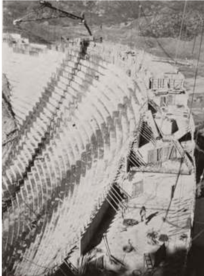
Figure 8. View of the main dam crest under construction, as seen from the left abutment crest. In this zone the shear key baffles were placed more frequently. Note how each step on the downstream face has a unique width, decreasing with upward elevation. Photo Lippincott Collection of U.C. Water Resources Center Archives.
