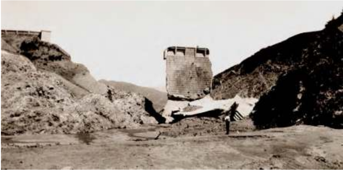
Figure 59. View looking upstream at the imposing monolith of Block 1. As in the previous photos, the gap between Block 5 and the chatter mark cut into Block 1 is noticeable, as is the clean character of the right abutment, swept clean of all debris in the later stages of the failure. Photo from the W.L. Huber Collection of the U.C. Water Resources Center Archives.
