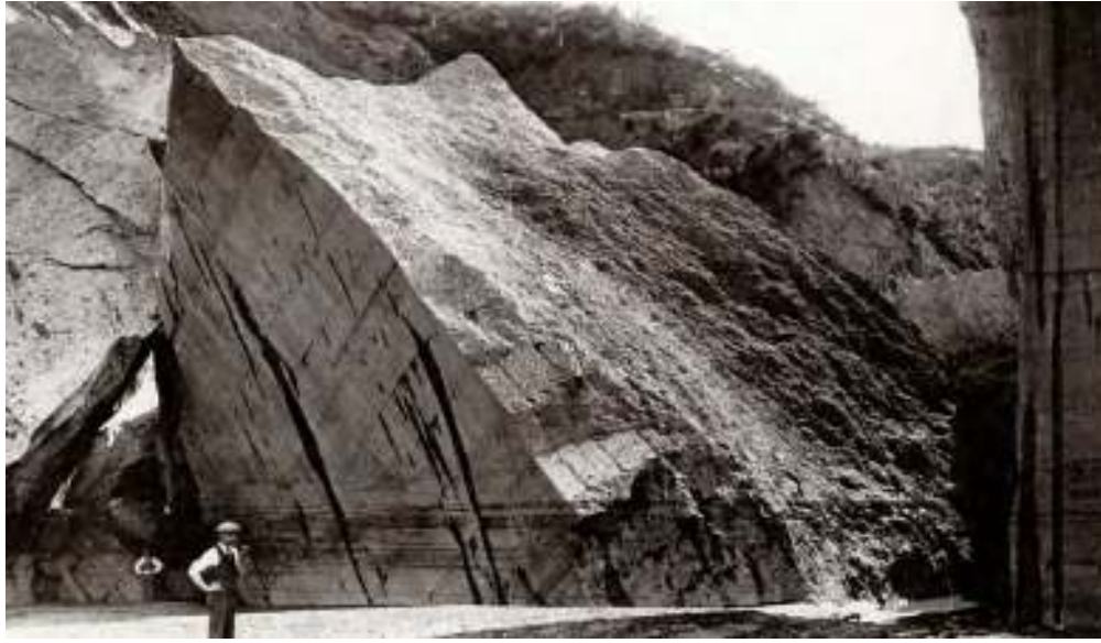
Figure 61. Ground view of Block 2 and a portion of 3, taken after the failure from upstream of Block 1. The horizontal scour marks across the inclined block testify to the reservoir stage when Block 2/3/4 toppled over. The reservoir was only about 17.5 feet deep, or nearly drained, when the left half of the dam's central core fell over. Photo from the W.L. Huber Collection of the U.C. Water Resources Center Archives.
