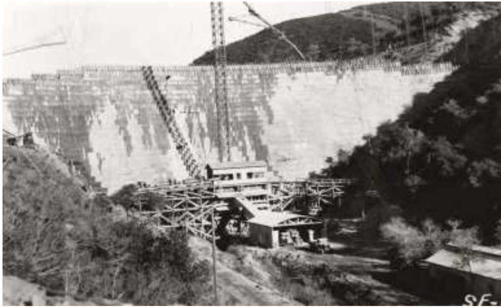
Figure 4 (Lower) - Same view as above, but about a year later, when the dam was nearing completion. Each of the steps were five feet high and forms can be seen along the upper three tiers. Note the dump trucks parked in the shed in front of the batch plant. Photo LA Dept of Water & Power.
