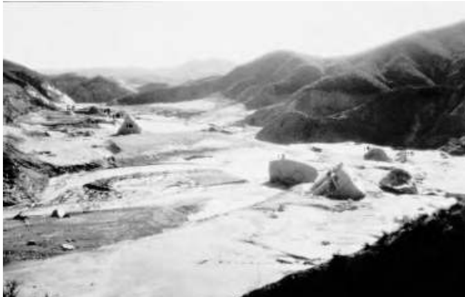
Figure 36. Displaced blocks of the dam, as viewed from a position about 1,000 feet downstream of the dam site. The block numbers written on the photo are those of the State Board of Inquiry (Fig. 38). Although Blocks 12 and 14 came from the base of the left abutment, they were situated between 22 and 26 feet higher than Block 16, seen further downstream and within the low flow channel.
