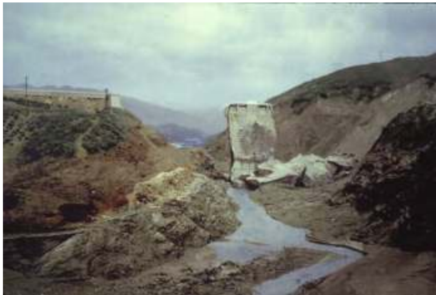
Figure 22. Upstream view of the dam site, taken within five days of the failure, when the downed power lines were still visible, leading into the left abutment landslide. Note position of the intact power poles high above the reservoir water line in background. Photo from C.H. Lee Collection, U.C. Water Resources Center Archives, colorized by Pony Horton.
