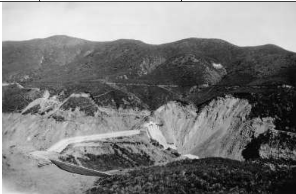
Figure 10 (lower). Same view taken after the failure. Note the prominent topographic bench in the Sierra Pelona escarpment, caused by massive landslipping. The east abutment slide is at right center. Another slump is obvious at left center, which dropped the old San Francisquito Cyn. Rd. about 50 feet (profiled in Fig. 45). From La Rue Collection at the Huntington Library.
