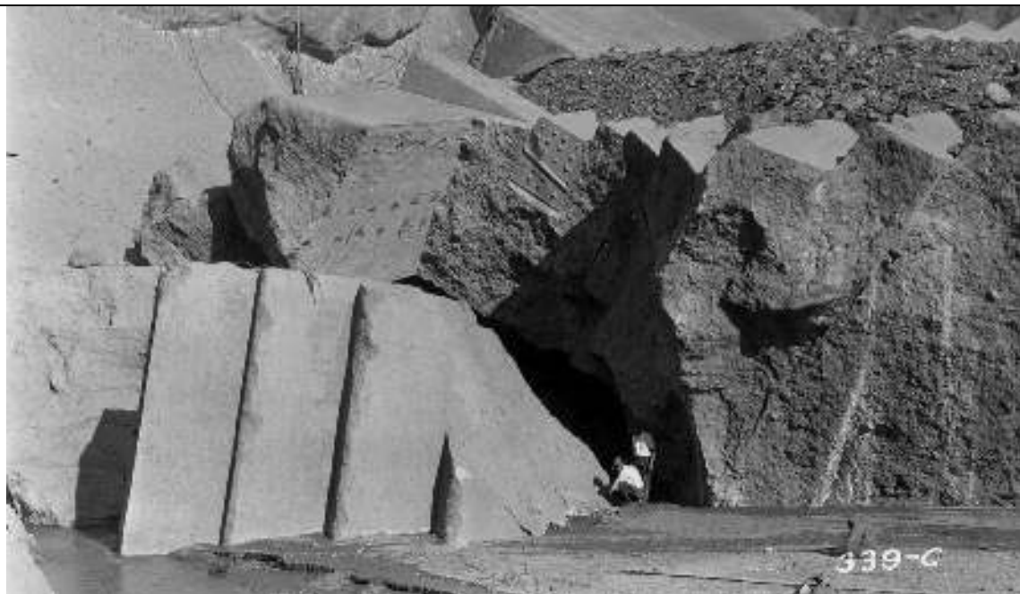
Figure 58. State survey party examining Block 6, which fell off of Block 5. Note the schist detritus infilling the 5 foot high steps of Block 5, 25 to 30 feet above the channel in foreground. Photo by H. Wildey, from author's collection.
