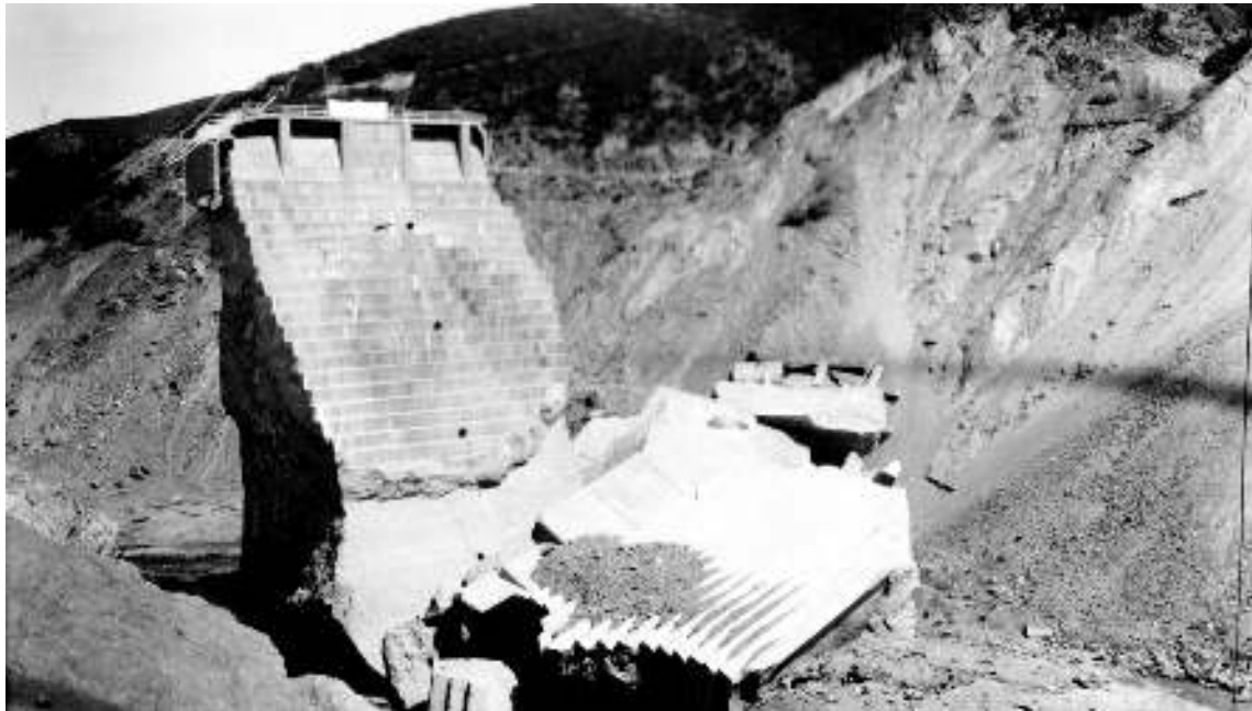
Figure 57. Upstream view of Block 5 sitting in front of Block 1 after the failure. Note the quantity of schist detritus sitting atop Block 5, testifying to its having been carried down slope in a slurry of disaggregated schist. Note the chatter marks on Block 1 cut by Block 5 and the latter's final resting position, about 30 feet lower. The material originally supporting Block 5 was likely swept away when the right abutment subsequently failed. Photo from the Lee collection, U.C. water Resources Center Archives.
