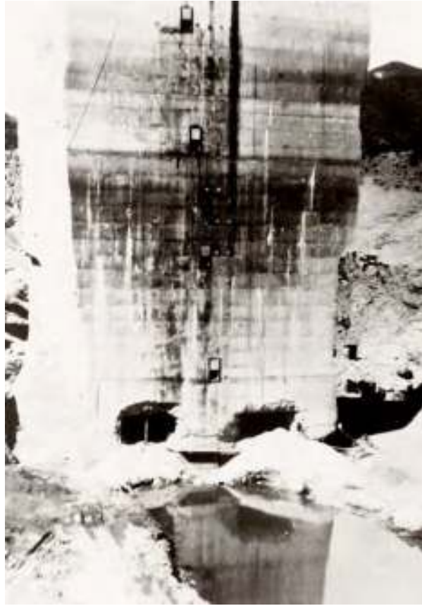
Figure 66. View looking at upstream heel of Block 1 in mid-1929, when the City was engaged in demolition work at the damsite. These adits in the upstream heel of Block 1 were loaded with dynamite and detonated, blowing the block backward, just like Blocks 2/3/4. Block 1 toppled backward and split into five discernable pieces. As in the case for Blocks 2/3/4, the concrete separated along undulatory cold pour joints, due to the weak tensile strength along these horizons, coated with a high water content laitance layer.
