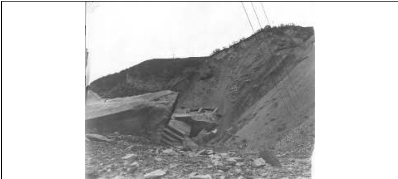
Figure 15. View looking upstream at the base of the left abutment landslide. Note the planar surface of Block 2, which broke along a cold pour joint. The three downed power lines clearly seen entering the slide area in this view had been clipped before the Governor's Board made their site inspection on March 22 nd . Note tandem SCE poles in distance, upstream of the east abutment landslide. Photo by H. Wildey, author's collection.
