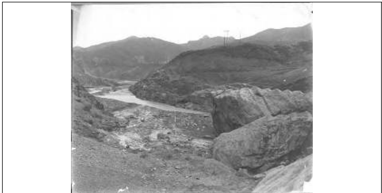
Figure 54. View from left abutment looking downstream at Block 7 wedged in behind Block 5. Note the accumulation of talus shed off the east abutment landslide scarp, which was 450 ft high. Photo by H. Wildey, from the author's collection.
