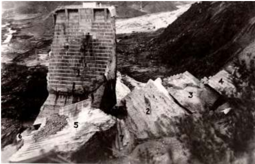
Figure 60. Upstream view of Blocks 1, 5 and 6 and those of Block 2, 3, 4, which rotated backward into a deep scour hole cut around the core's left side. Note the broken surface of Block 2 and most of Block 3, where the dam's downstream steps have been sheared off. Historian Charles Outland unravelled this puzzle while he was writing Man Made Disaster in the early 1960s. Photo from L.A. Dept. of Water & Power.
