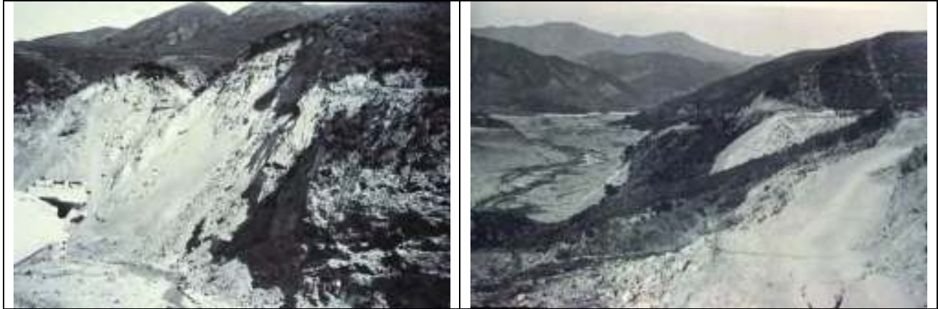
Figure 45. Left photo shows exposed scarp of the east abutment landslide extending well above old San Francisquito Cyn. Rd. Image at right shows gross ground deformations along the Bee Highline Road, about 300 feet above the dam's left abutment. The slope dropped two to nine feet above the east abutment slide. Both photos from Ventura County Museum of History & Art.
