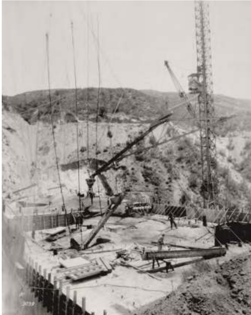
Figure 7. View looking west southwest towards the left abutment, in the Pelona Schist. Excavation of about 20 feet of schist can be seen, as well as the planar nature of the foliation surface, paralleling the abutment. Note the standing ponds of laitance moisture sitting upon the concrete pillows in foreground. Photo from L.A. Dept. of Water and Power.
