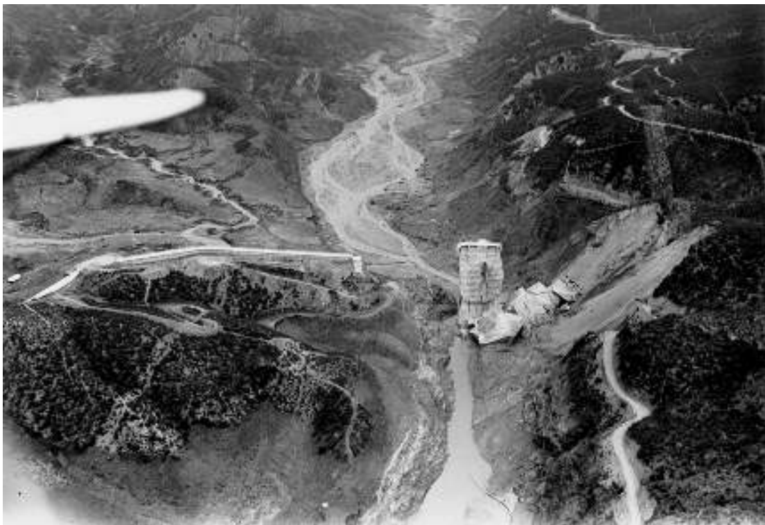
Figure 29. Aerial oblique view looking upstream at the dam area the morning after the failure. Note how high the east abutment landslide extended above the reservoir. Also, note the massive slump block upstream of the dam, caused by rapid drawdown (UCLA Spence Photo Collection).
