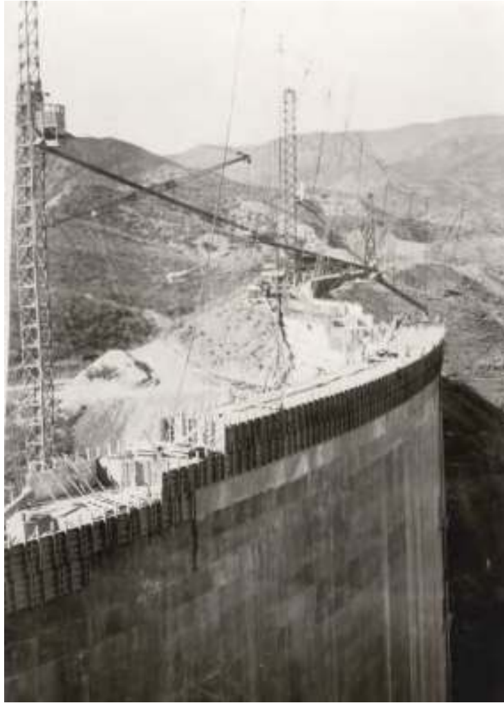
Figure 9. The dam design was amended to increase the overall height by 20 feet, taken in 10-foot increases on two occasions, a year apart. This view shows the dam topping out, sometime in 1926. The finished crest width was 16 feet. By this time the contractor was forced to install additional towers to aid in concrete placement along the dike section in the background. Photo from Lippincott Collection of U.C. Water Resources Center Archives.
