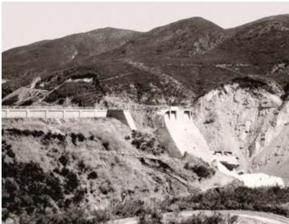
Figure 62. Ground view of the right abutment, just downstream of the dam following the failure. The intact nature of all vegetation on the dam's right abutment to an elevation at least 75 feet below the dam's crest suggests that the reservoir was 2/3 drained before the right abutment of the dam gave way (also see Fig. 29).
