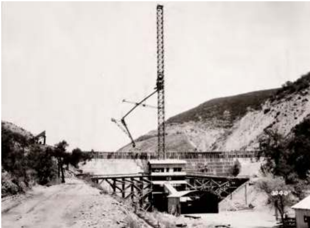
Figure 4 (upper). Upstream view of St. Francis Dam under construction, in the fall of 1924. The contractor’s concrete batch plant lies in front of the dam. The large shed in front of this structure was where aggregate collected down-canyon was end dumped into the plant. Photo from the Lippincott collection, U.C. Water Resources Center Archives.
