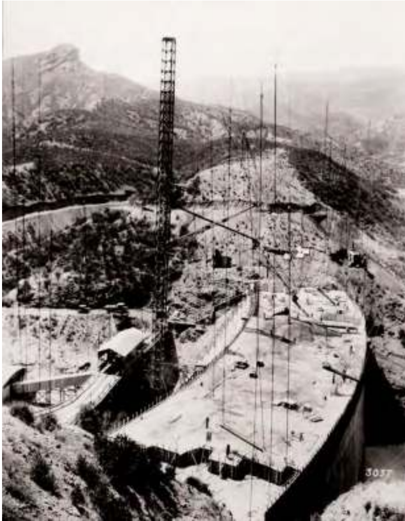
Figure 5. View looking northwest towards the left abutment, during the dam's construction, around March 1925. Shear key baffles are being placed within the dam, about 50 and 100 feet from either abutment. Note the steam shovel working on the right abutment and the contractor's tower, used to deliver concrete to the central dam area via a system of cables.
