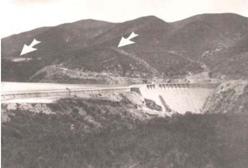
Figure 10 (upper). Part of a three photo panorama, believed to have been imaged in the spring of 1927, when the reservoir was about 20 feet below the spillway slits. Note the position of San Francisquito Canyon Road, cutting across the dam's left abutment, about 13 feet above crest. Also note the prominent terrace platforms exposed in the Pelona schist. Photo L.A. Dept. of Water & Power.
