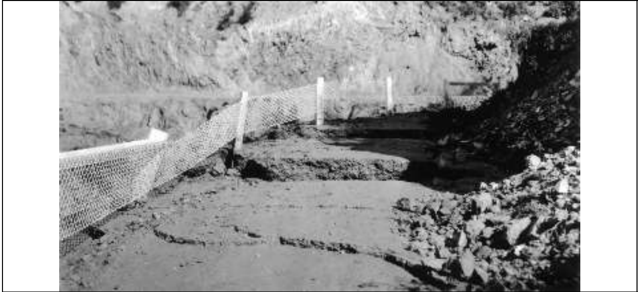
Fig. 11 - En-echelon tension cracks in San Francisquito Canyon Road several hundred feet upstream and about 20 feet above the dam's left abutment. The Ray Silvey family noted that one of these scarps was 12 inches high when they passed the dam between 8:30 and 9 PM, forcing them to stop their car and excavate ramps for their tires. These scarps were developed in the Pelona Schist. Photo by Bailey Willis, from the St. Francis Dam Disaster Collection at the Huntington Library.
