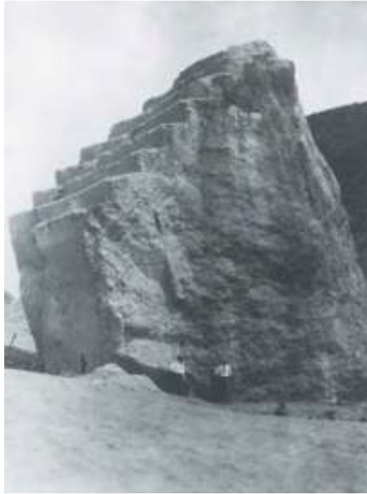
Figure 37. Close-up view of Block 16 (State designation) or 44 (BWWS designation), at 10,000 tons, the largest of the dam's displaced blocks. It was found about 1,500 feet downstream of the dam. The only plausible mechanism by which such a large block could be hydraulically transported would be by saltation in a dense slurry, akin to a massive debris flow. Photo from the Lee Collection, U.C. Water Resources Center Archives.
