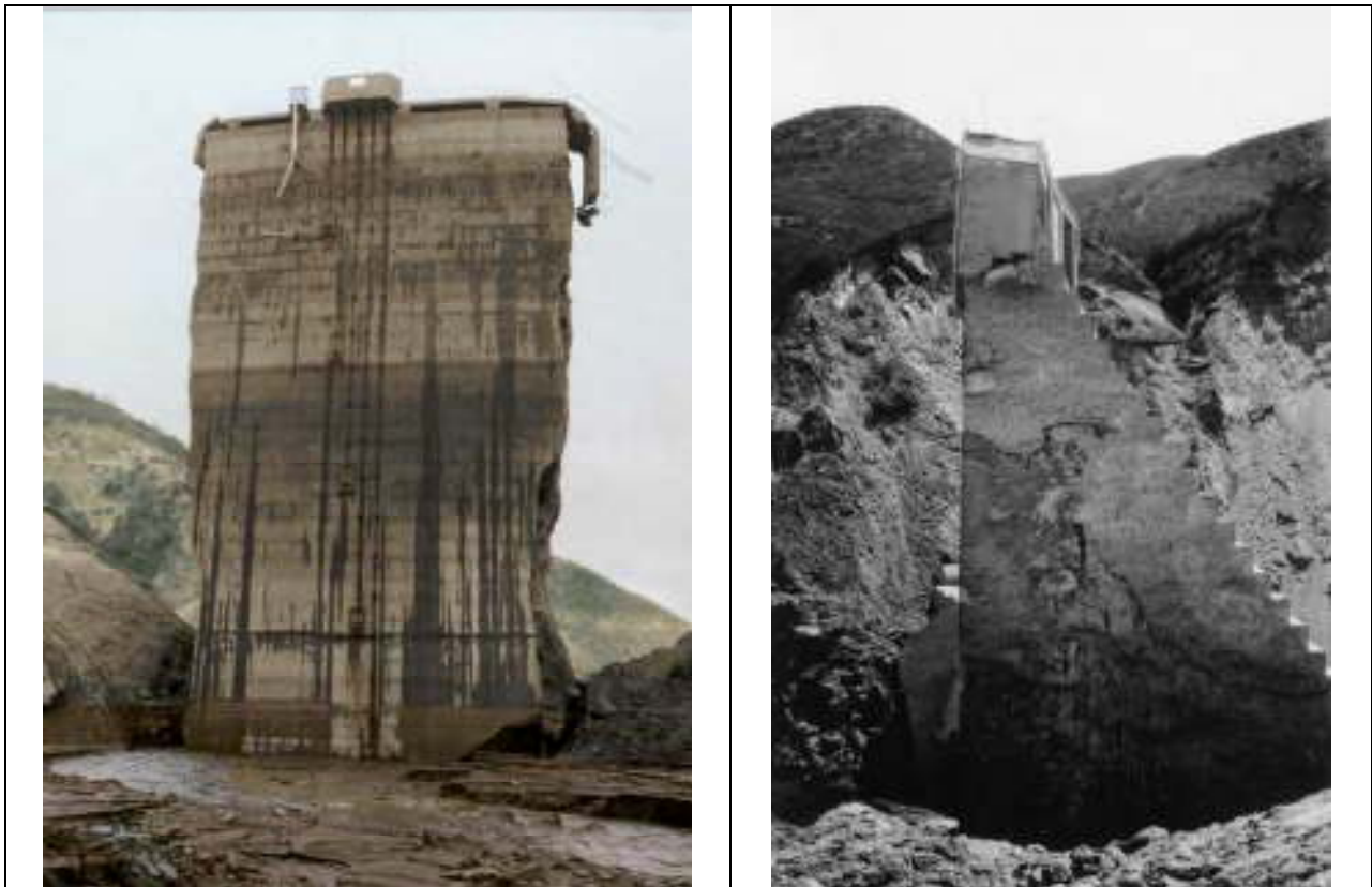
Figure 17. Left - Carl Grunsky discovered the gage attendant's wooden ladder wedged inside an enormous tension crack in the right upstream heel of Block 1 (from Ventura County Museum of History & Art; colorized by Pony Horton). Right – Profile view of the Block 1 monolith. No discernable upstream batter can be seen near elevation 1730, about half the height of the block (from La Rue Collection of the Huntington Library ).
