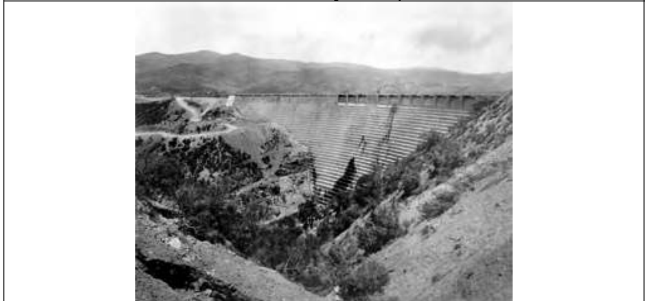
Figure 2 – St. Francis Dam as viewed from the old road, from the left abutment. The old access road with the 18% grade can be seen climbing the right abutment, below the dike. This was where the ‘muddy water’ was observed by damkeeper Harnishfaeger on the morning of the failure. Also note how it would be difficult to notice people with flashlights at the base of the dam’s left abutment, which cannot be seen from the old road.
