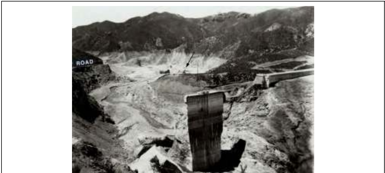
Figure 14. Downstream view of the dam site after the failure, showing location of the SCE 70 Kv Borel Power Line poles, about 60 feet above the high water mark on the right abutment, about 650 feet downstream of the dam. Photo from Ventura County Museum of History and Art.
