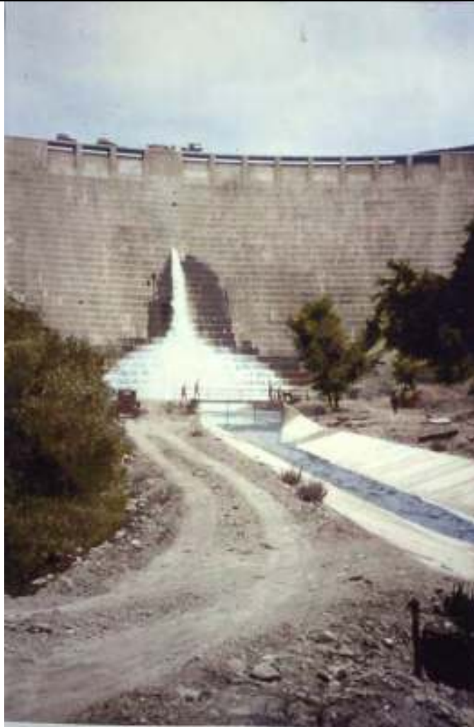
Figure 12. Frontal elevation view of St. Francis Dam, believed to be taken the day of dedication, in May 1926. Note the eleven crest spillway bays, each only 18 inches high, and the concrete-lined trapezoidal channel in foreground, which ran 7,300 feet downstream, to Powerhouse 2. Image colorized by Pony Horton.
